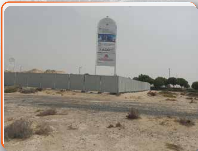
RESIDENTIAL BUILDING GROUND + 4TYPICAL+ROOF+SERVICES+ BOUNDARY WALL AT PLOT NO. RB-58 RESIDENTIAL CITY AT DUBAI SOUTH DUBAI, U.A.E
