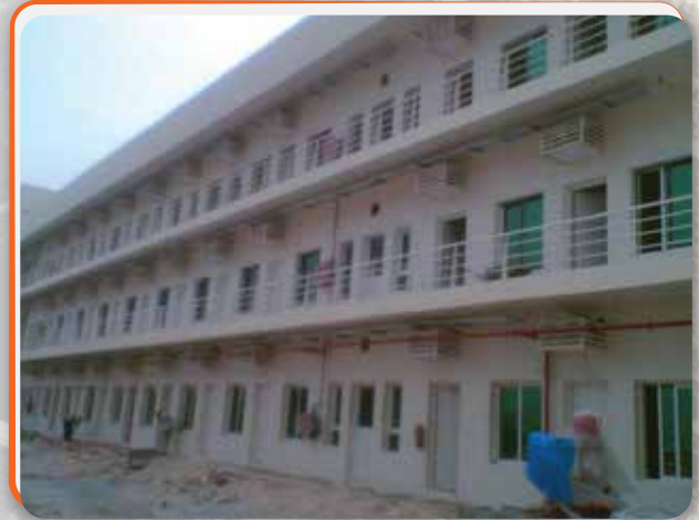
CONCEPT ENGINEERING CONSULTANTS P-04 G+2 LABOUR ACCOMODATION IN AL QUOZ AREA DUBAI. FOR MR. HASAN AL FALASI
