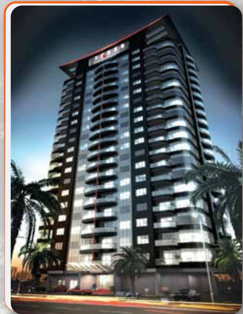
LAMBORGHINI RESIDENCE TOWER IN DUBAI SPORTS CITY
